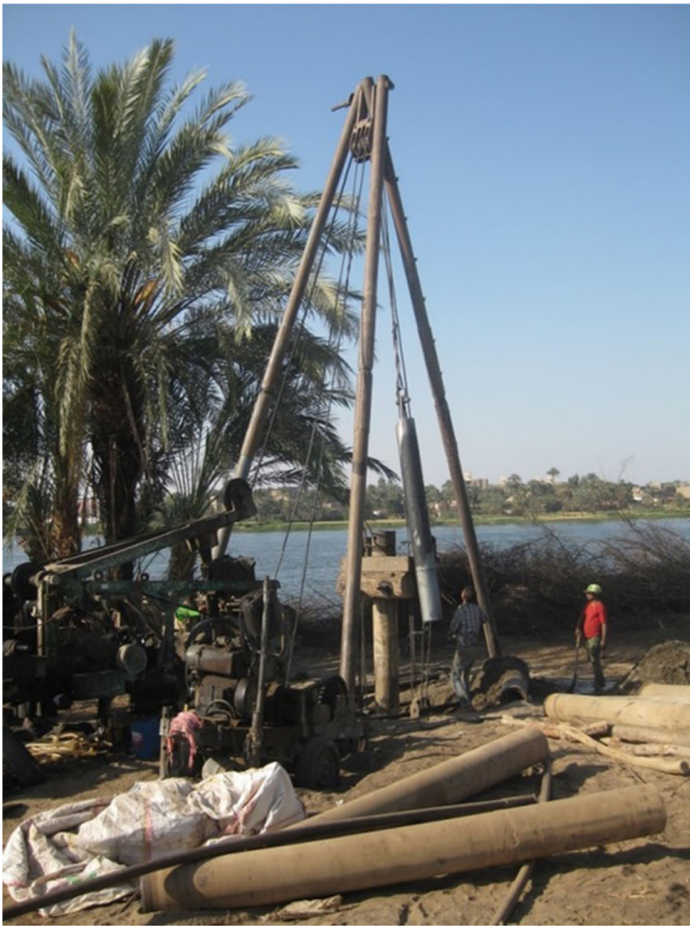
Fig. 7 Drilling of riverbank filtration wells at the Nile River, Luxor, Egypt, March 2018. Seasonal low river water level, frequent spills of oil and other pollutants and high turbidity during high flow cause problems in surface-water abstraction and subsequent treatment. A short distance between the abstraction wells and the river bank is sufficient to remove particles, to buffer spills and to ensure a high portion of bank filtrate and a low portion of manganese-rich land-side groundwater (Photograph courtesy of T. Grischek, University of Applied Sciences Dresden, HTWD)
